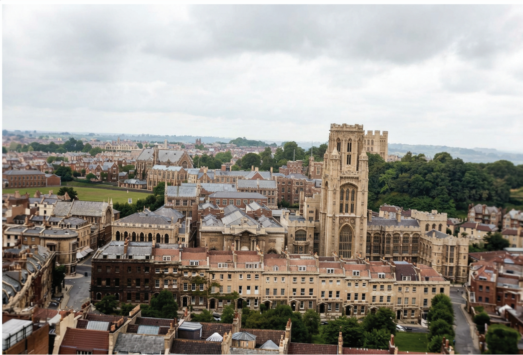
Bristol, c1933, from Cabot Tower - looking North East. The prominent structure is Wills Memorial Building.
